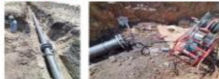
Pipe Welding & Pressure Testing
