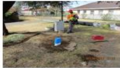
Installation of water meters
