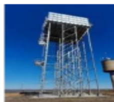
Newly Constructed Elevated Tower
