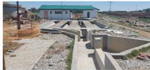
Inlet Works – Concrete repairs (19/10/2023)
